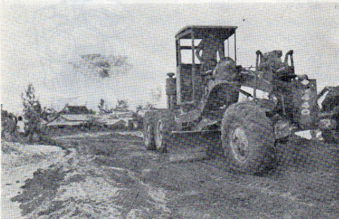
At a by-pass road at the Vietnamese Amputee Hospital near Camp Tien Sha, a 53 heavy equipment operator uses his grader to level the surface.
