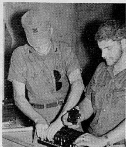
R.D. WHITEHEAD CE2 AND H.T. LUNDGREN CEW3 ASSEMBLING A CIRCUIT BREAKER PANEL.
