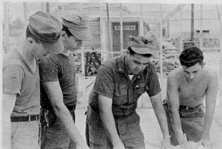
C.E. GENTRY CEW2 GOING OVER PLANS OF WIRING FOR PROJECT AT NSA HOSPITAL WITH W.N. SOUER CEP3, J.R. CURTIS CN, D.J. MAGYAR CN.
