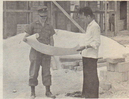
CHAPLAIN FIOLE AND FATHER NHAN LOOK OVER PLANS FOR 8 ROOM SCHOOL, IN AN CU III REFUGEE VILLAGE, THAT MCB-53 CIVIC ACTION IS HELPING TO BUILD.
