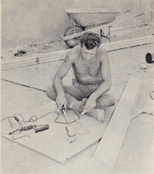
SW3 W. SHKAPITCH LEADING DOWNSPOUT FOR THE GENERALS QUARTERS.
