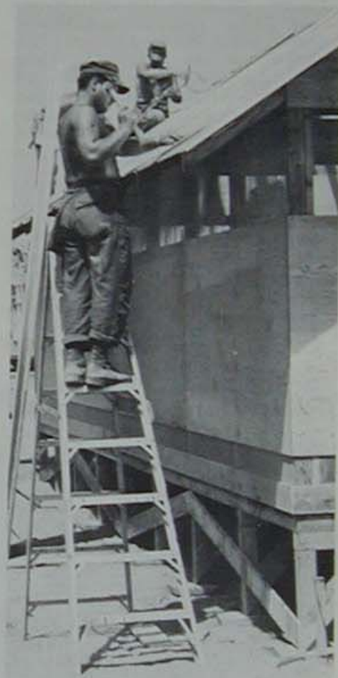
A builder hammers down the final section of roofing on a hut while two CEs rig up the wiring.
